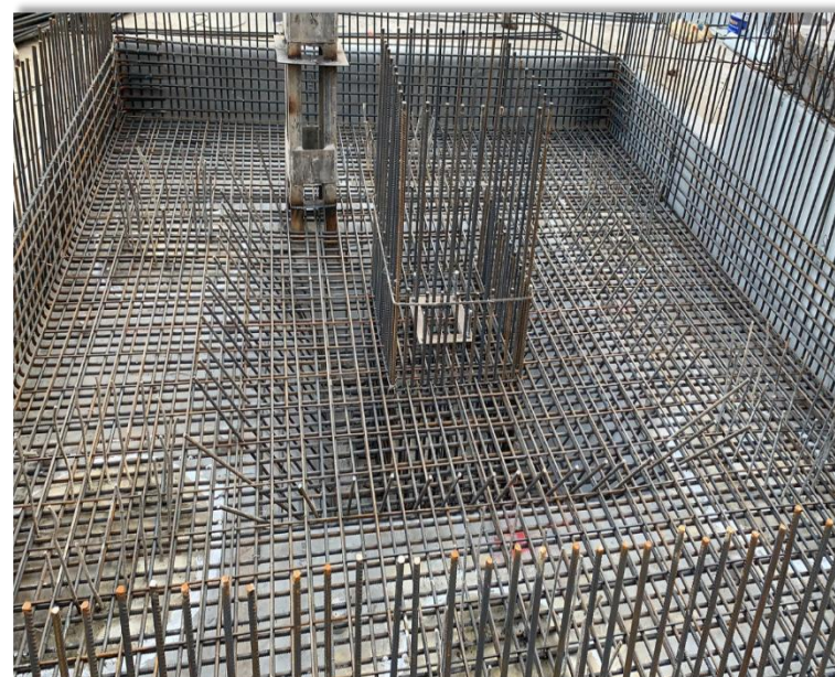
钢铁柱基坑地脚螺栓预埋样
